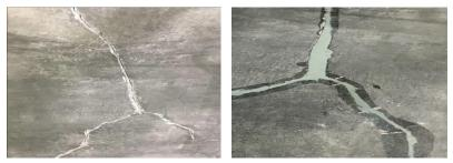
**CM2 MIXING INSTRUCTIONS: CM2** is a fast cure product Mix "**Part A**" and "**Part B**" in equal parts (1:1) by volume. Only mix 4-6 oz of each part at a time, mixing a total of 8-12 ounces. Pour each part into squeeze bottle or similar applicator and vigorously shake for 10-12 seconds. Immediately use as the product will begin to cure within 10 minutes, temperature dependent.
