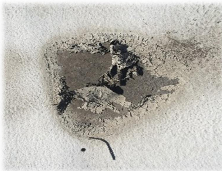
Remove Degraded Coating
