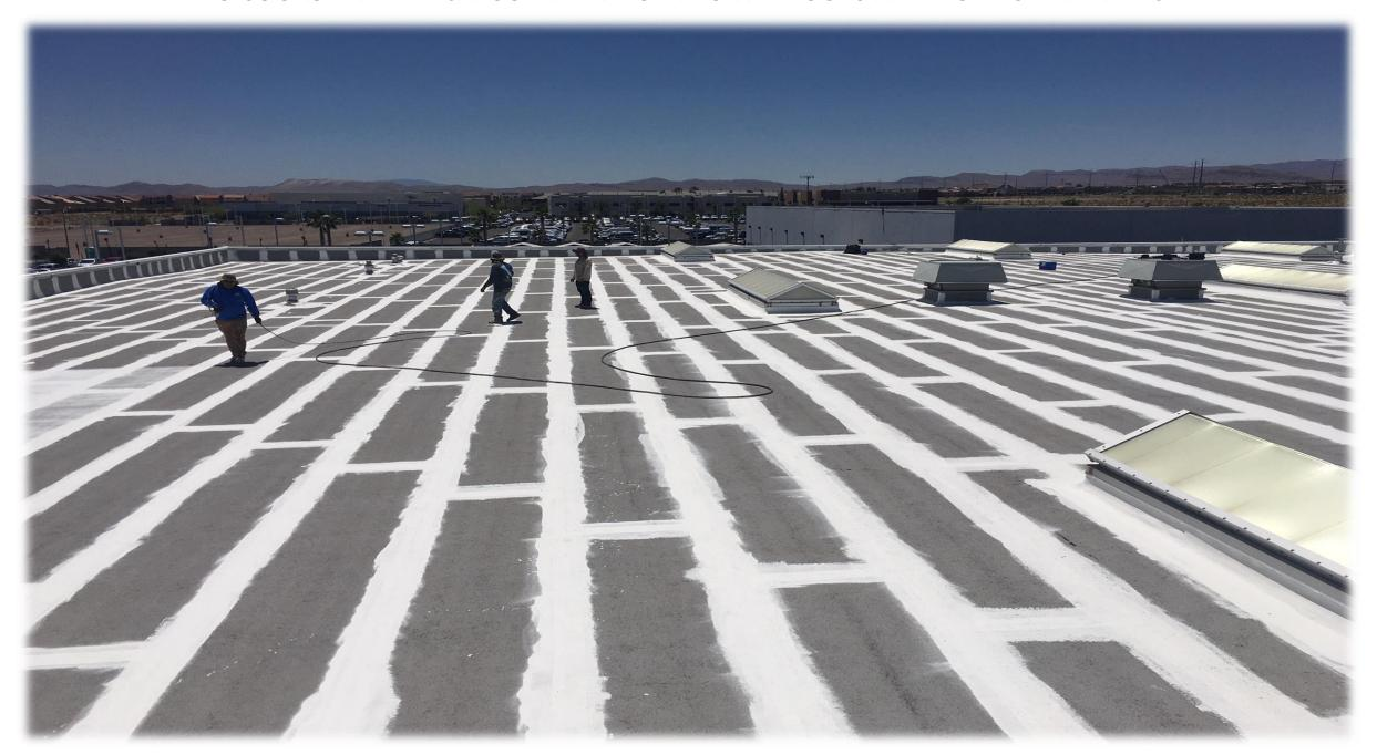
APPLY SG40 BASECOAT TO THE ROOF DECK AND OVER THE SEAMS
