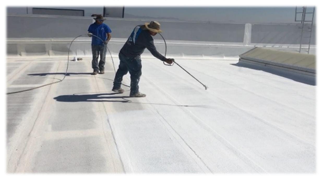
SG40 BASECOAT / SG54 TOPCOAT PROVIDE HIGH ADHESION, HIGH WATER RESISTANCE / SYSTEM COMPATIBILITY
