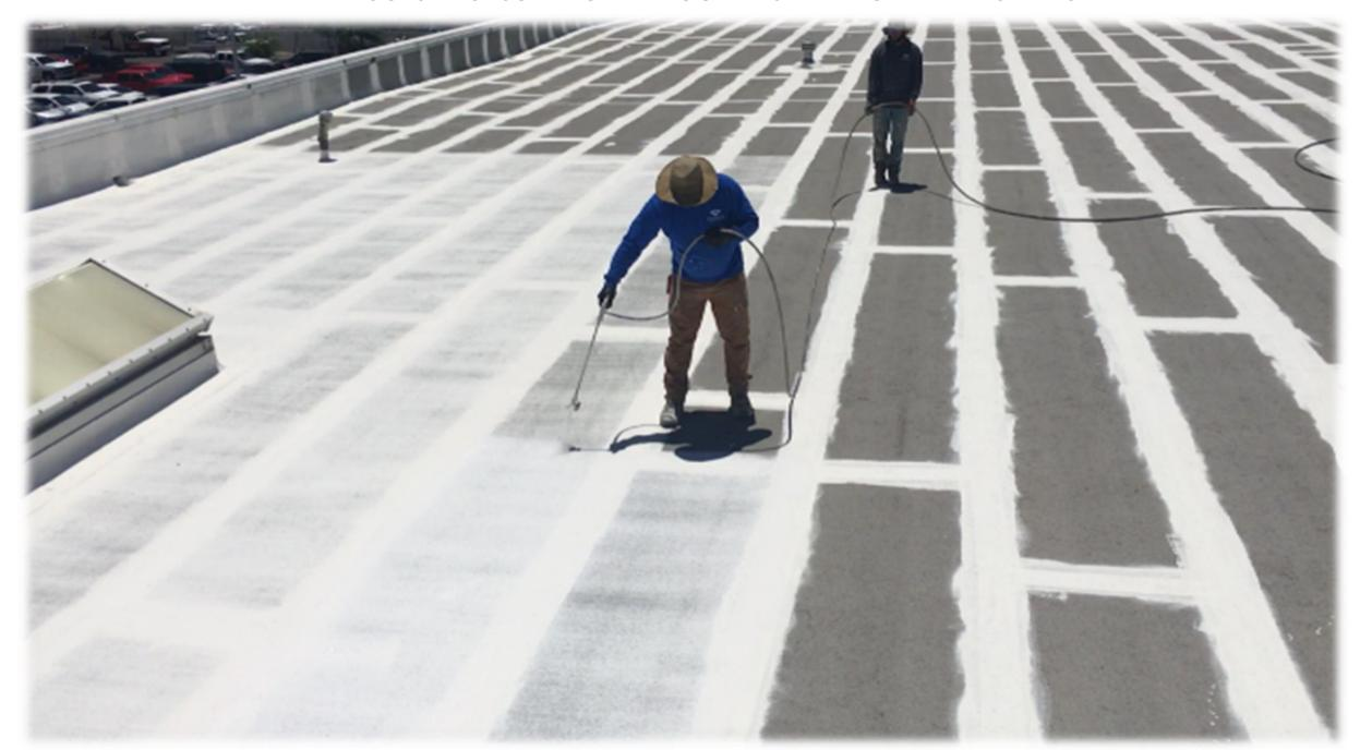
SG40 BASECOAT APPLIED AT 2.5 GALLONS PER SQUARE OVER THE SEAMS AND THE ENTIRE ROOF DECK
